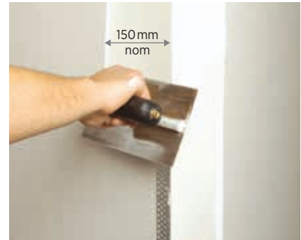
2. Apply first coat to both corner faces
