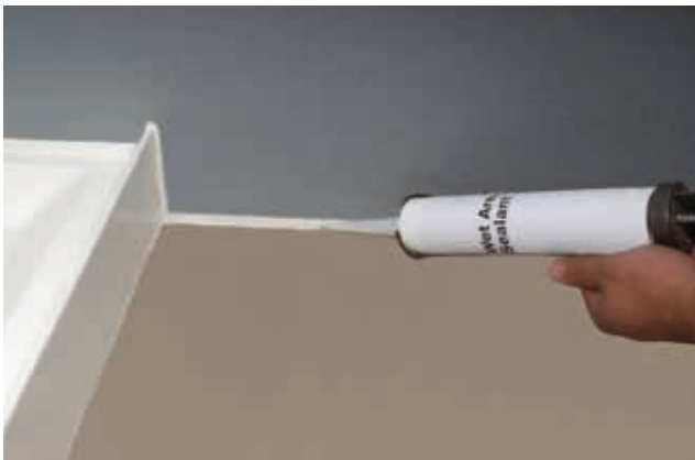
Figure 60: Seal Floor and Wall Junctions
