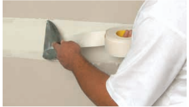
2. First coat - Bed tape
