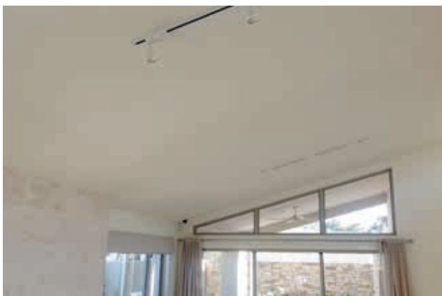
Figure 5: Plasterboard surface under normal lighting conditions
