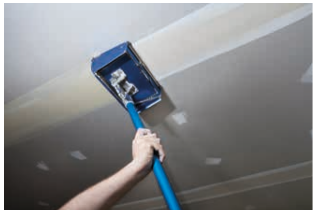
Figure 86: Flat Box Application
