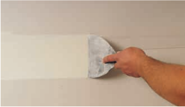
1. First coat - Bedding compound
