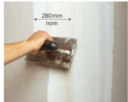
4. Apply third coat to corner faces
